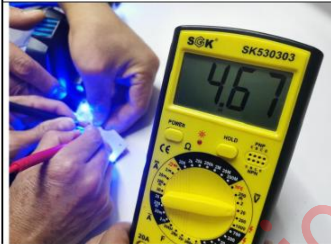
Led light working voltage check
